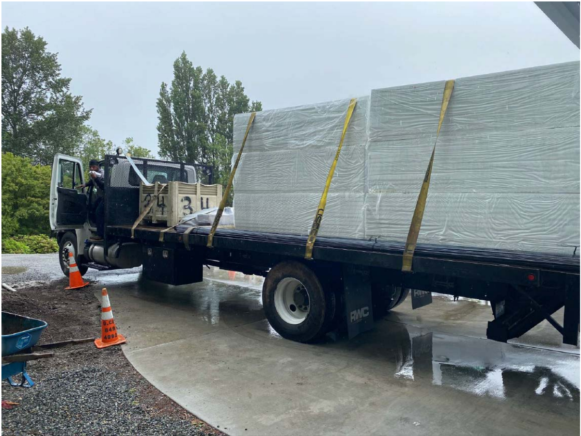
This photograph shows a truck delivering construction materials to the Yangs' residence. The truck hit the gutter on the Niedermans' garage and nearly hit the garage door.
